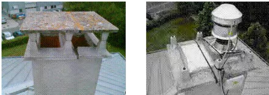
Photo 3: Basic extractor and static extractor
