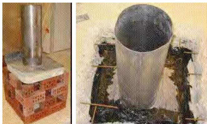
Photo 2: Installing new sump for natural depressurisation
