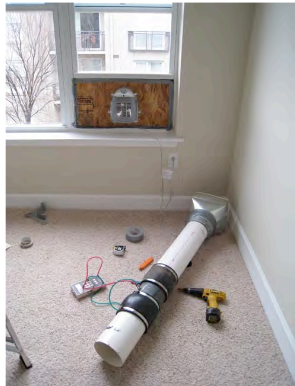
Figure 10 Combination ventilation fan and heater with calibrated flow grid airflow measuring setup
