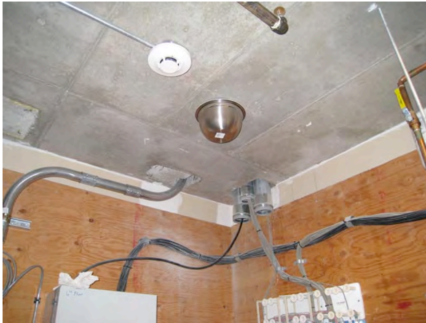
Figure 5 E-PERM Emanation of ceiling of electrical room
