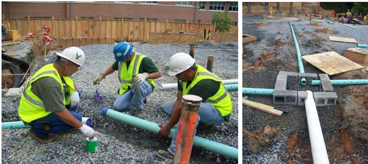
Figure 2: Connecting Isolated Slab Areas with a Central Plenum Box
