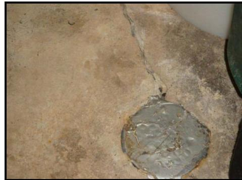
Photograph 2- Temporarily Covered Sump Hole
