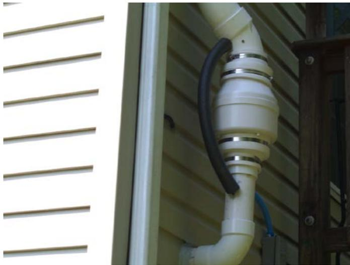
Figure 3 – Diverta Drain Installed
