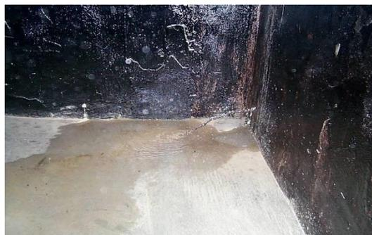
Figure (2) Failure of bitumen waterproofing system in basement
