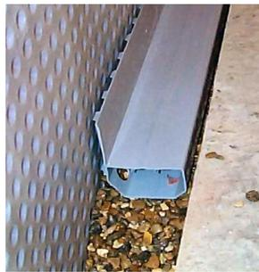
Figure (8) Typical perimeter drainage channel
