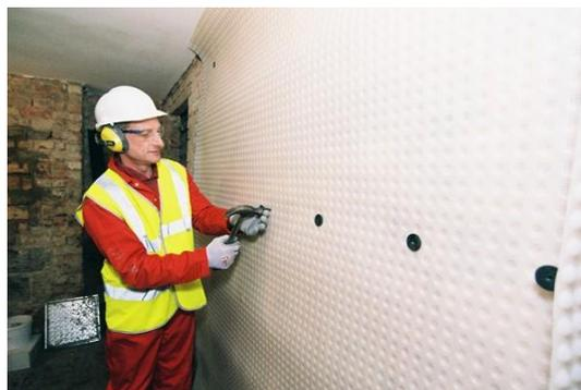
Figure (6) Membrane plug fixings
