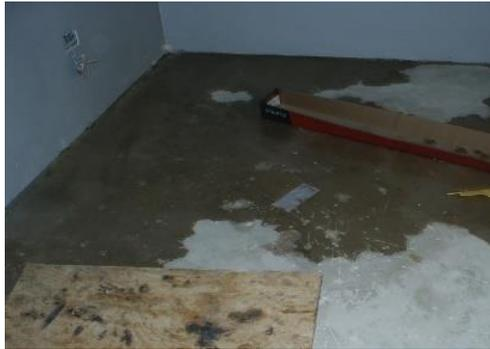
Figure (3) Failure of newbuild waterproofing system in basement
