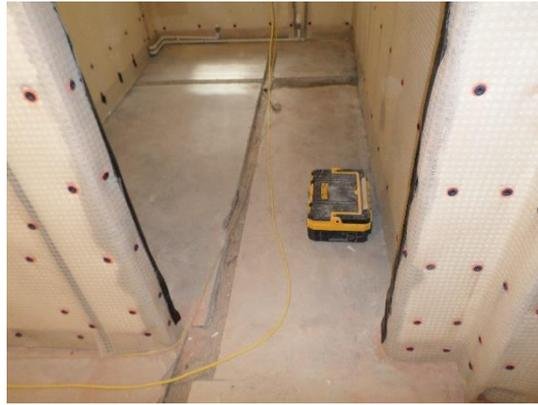
Figure (7) Membrane taped joints
