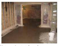
Not wanting to take a chance on anything, we also decided to seal the floor with radon seal before the new floor coverings are installed. (Better safe than sorry.) After the work was done we had to replace everything, even the tile floor in the bathroom.
