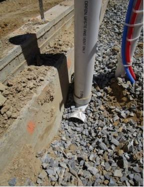
Extending the Tee Fitting with perforated pipe prevents closure of the suction point. This is a minimal cost to the builder.
