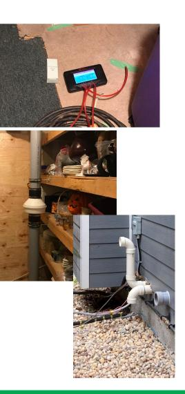
Require proper radon diagnostics and design as part of the installation of our mitigation systems to mitigate the entire footprint of the building.
