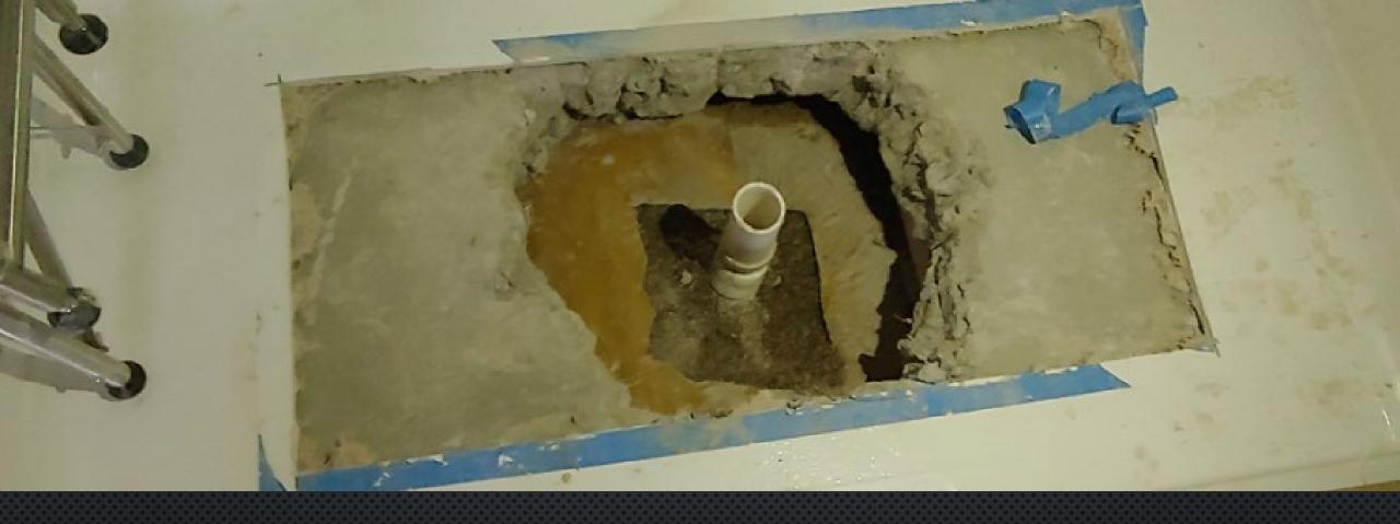
THE PLUMBER CUT THE VAPOR BARRIER FOR 42 SHOWER PANS DUE TO MEASUREMENT ISSUES. WE DID NOT FIND OUT UNTIL 3 WEEKS BEFORE THE PROJECT COMPLETION. EVERY DRAIN HAD TO BE EXPOSED AND REPAIRED.
