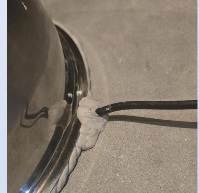
Use extra Mortite for sealing around the opening and cord
