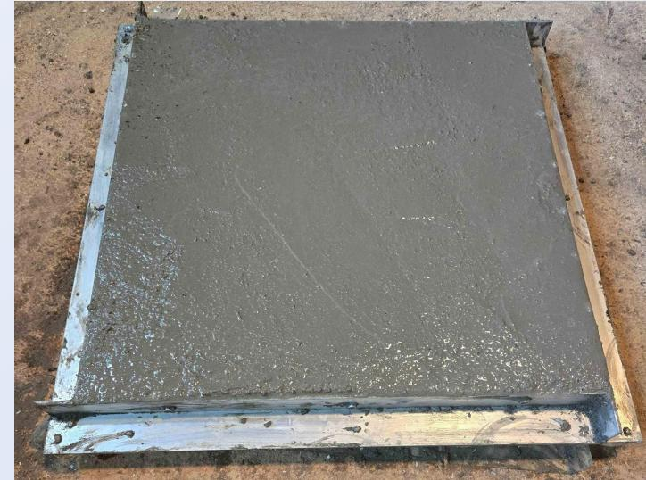
After the Concrete set, the  $\frac{3}{4}$ " plywood was removed from the bottom
