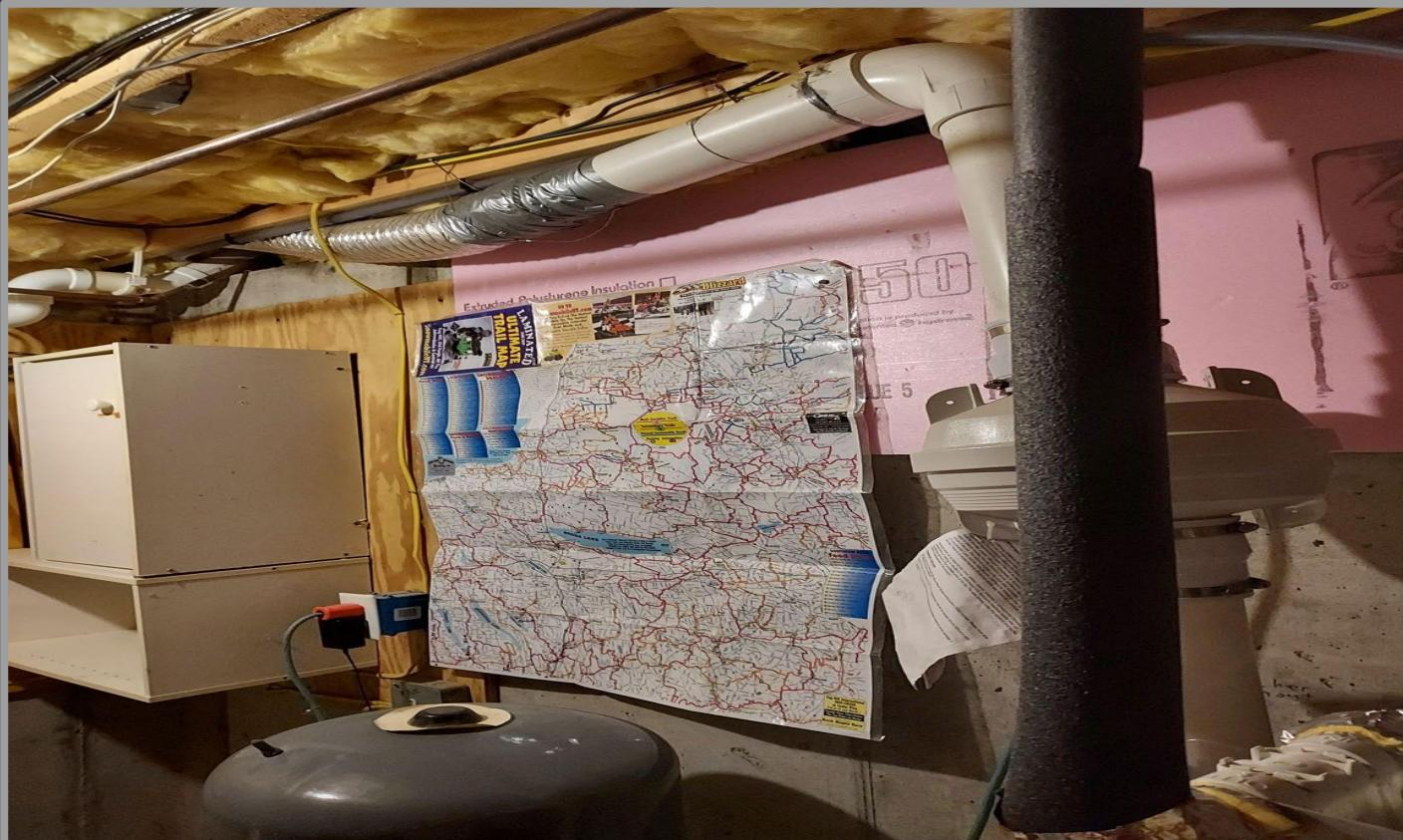
Fan on the interior goes from PVC to Flex Metal dryer vent
