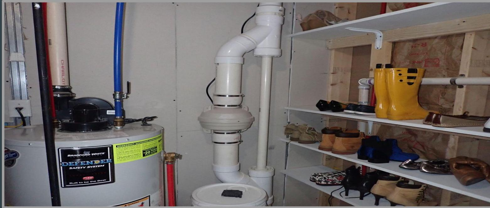
The system vented into the second floor joist, it never went to the exterior.
